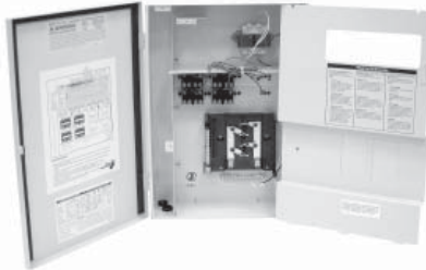
6614 Sub-Panel Power Center (with mounting brackets)
